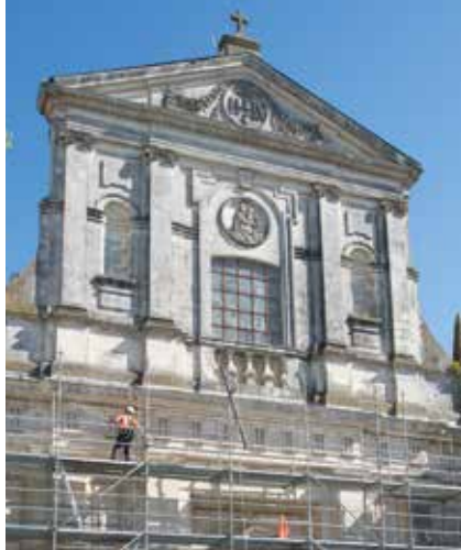
Restauration façade sud
